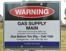
Pipeline markers do not show the exact location of a pipeline but will typically be located on both sides of public roads, railways, rivers, vehicle tracks, or property boundaries, and are generally installed along the route of a transmission pipeline's right-of-way or easement, which can range from 6 to 25 metres wide.
