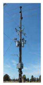
Figure 14: New generation SWER ACR (pictured on the right hand side of the pole)
