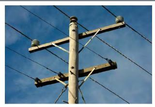
Figure 18: Power pole with high voltage lines at the top of the pole and low voltage lines underneath
