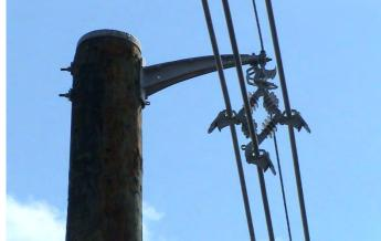
Figure 23: Covered wire with support wire
