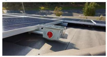
Figure 3: A rooftop DC isolator installed next to solar panels with shroud (protective cover)
