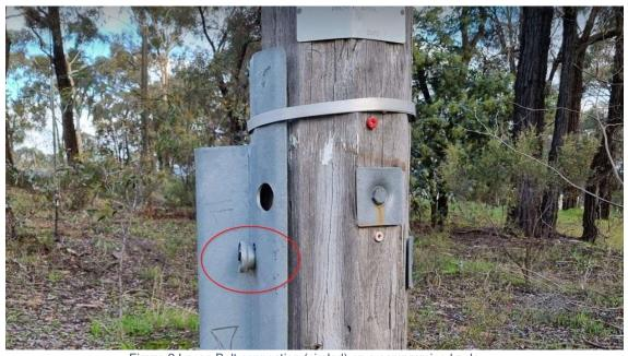
Figure 2 Loose Bolt connection (circled) on a compromised pole Note: outer fibres compress inwards – reducing the effectiveness and strength of the pole / reinforcement connection
