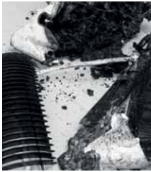
A burned out heater.
